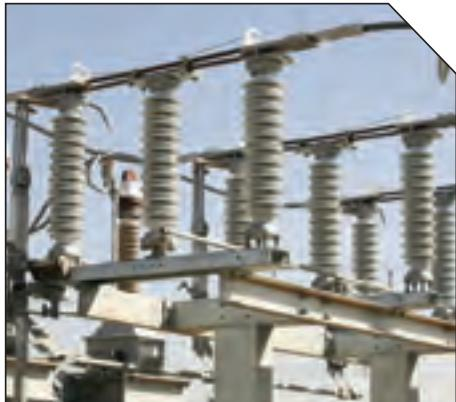
The AEM type High Voltage (HV) Double Break Disconnectors are designed for outdoor transmission substation isolation duty in power transmission networks.
