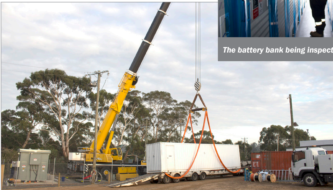
Crews install the containerized PureWave® Storage Management System.
