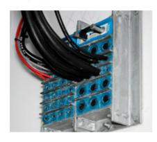
over the plant as well as under the raised floor in the switching room: "The best thing with the Roxtec system in comparison with other methods is that we can seal many cables in each opening. We save a lot of time by routing the cables first and sealing them afterwards." The seals also provide spare capacity for further environmental efforts. Download pdf.
